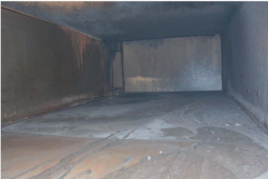
Figure 6 Picture inside the duct after installed AirMaid (January 2011).
